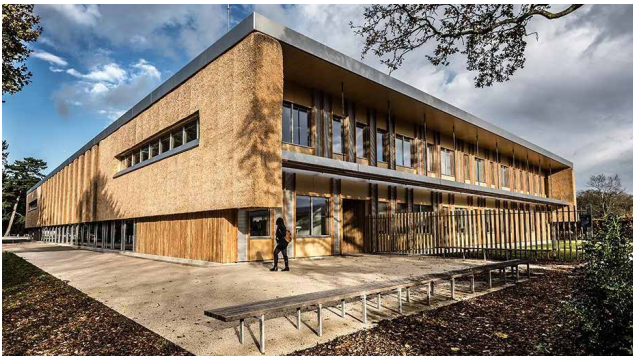
Figure 1.13 - The Enterprise Centre Source: Architype
